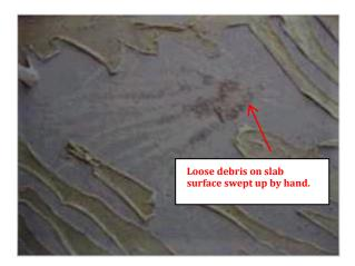
Failure – Vinyl bubbling/lifting away from slab.
