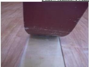
Failure – planks lifting at corners and sides.
