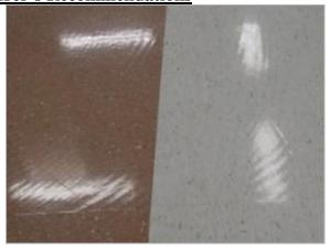
Failure – Ridges visible in flooring. Inspection Findings – Rolling floor after install did not flatten out adhesive trowel marks.
